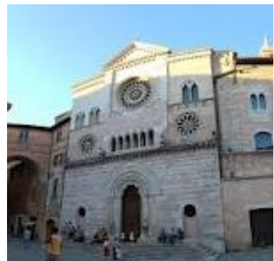
DUOMO Foligno (PG) Consolidamento e restauro Cripta
