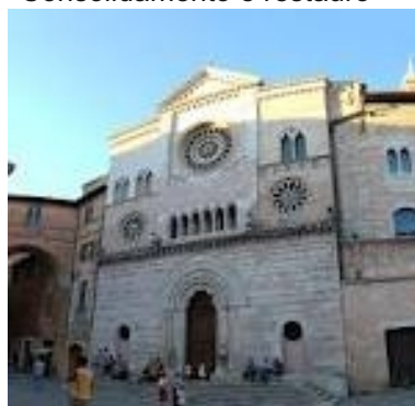
DUOMO Foligno (PG) Consolidamento e restauro Cripta
